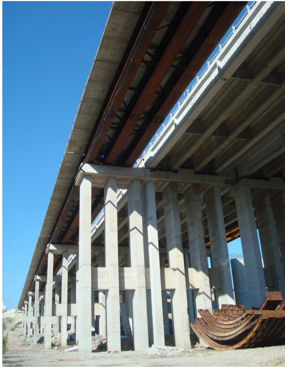
Fig. 1: Widening intervention of Morignano Viaduct
